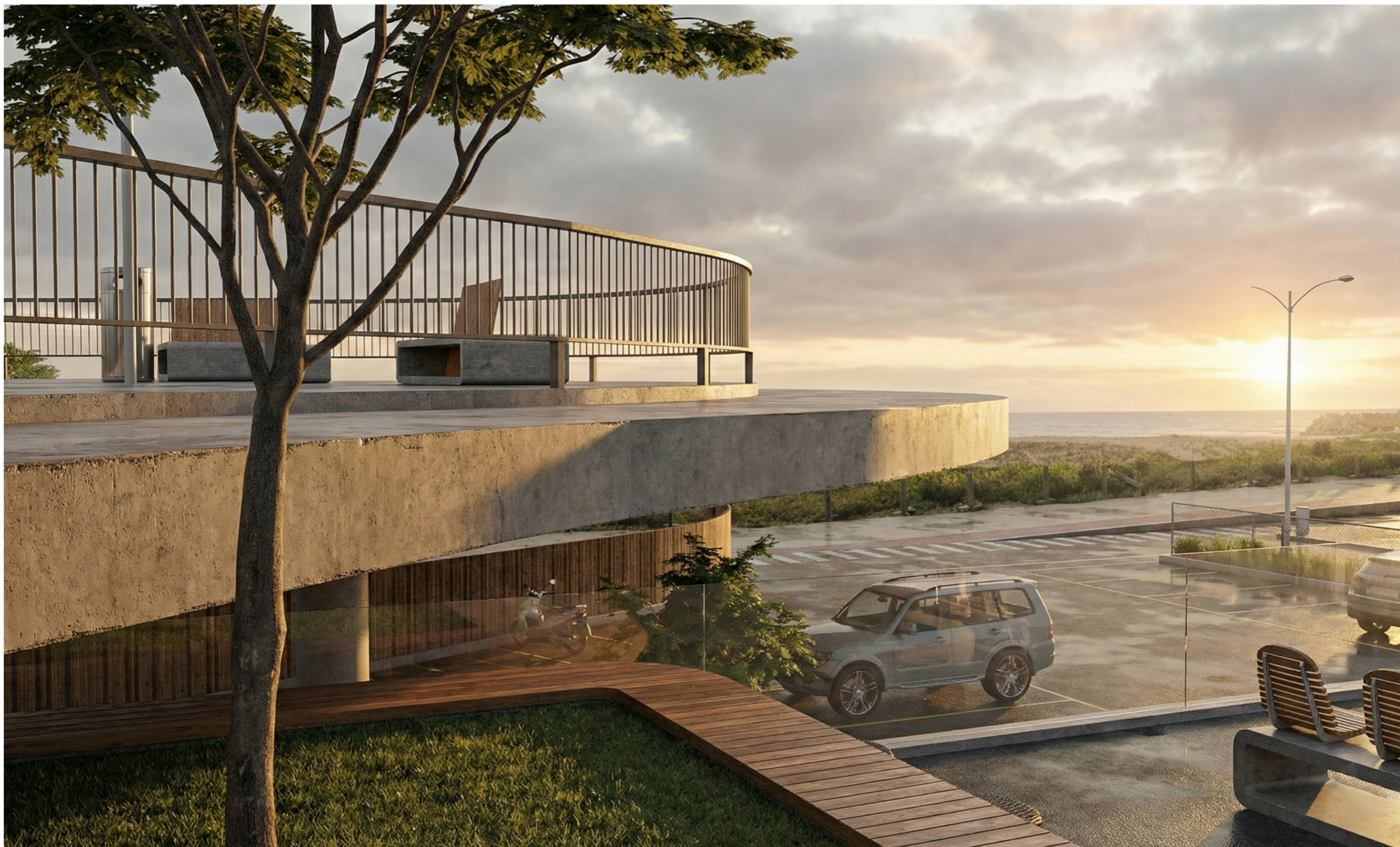
Vista do rooftop
